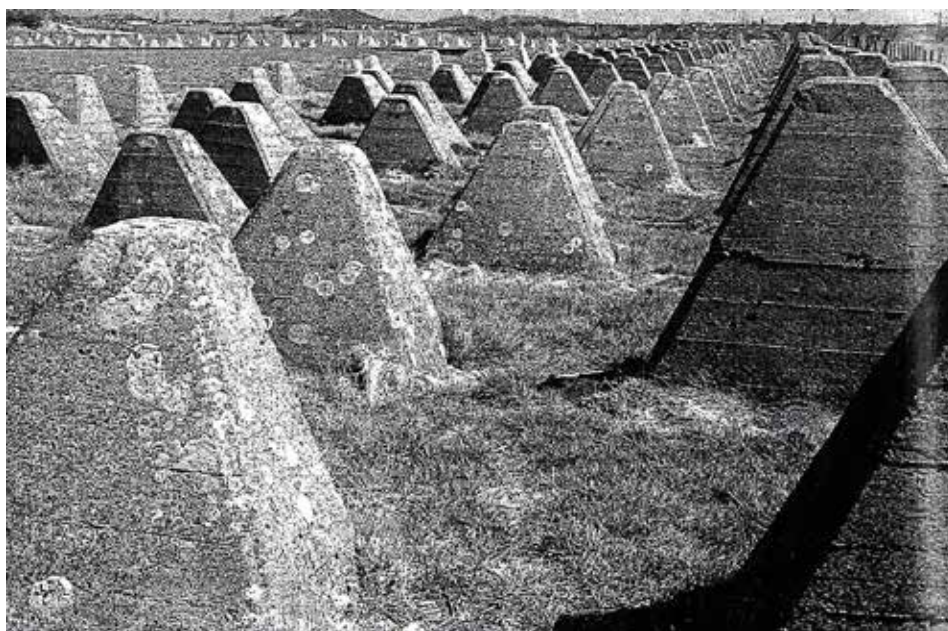
Figure 4. Part of the so-called Siegfried Line in Germany near the Dutch and Belgian border. These concrete structures known as "dragon's teeth" were designed to block the passage of tanks (Wegener 2006:282).
