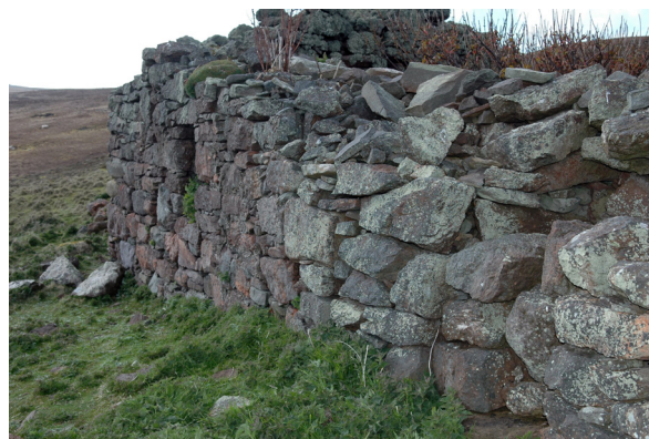
Illus. 22 South wall of Tulloch's Bød showing the contrast in masonry between the coursed west side (background) and the reduced door and east jamb (foreground).
