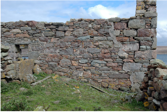
Illus. 12 South end of exterior of west wall showing break in fabric between the wall and gable end.
