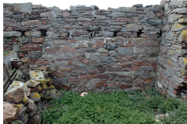
Illus. 13 Inside of west wall looking west. There is a clear distinction between the larger stones below the joist holes and the stones above.
